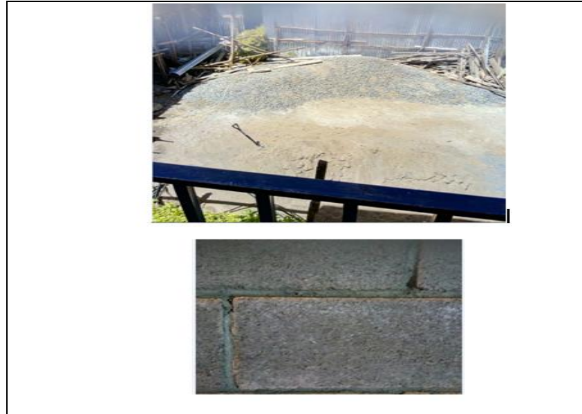
Figure A2: A photo of Sampling Building Materials in the Field
